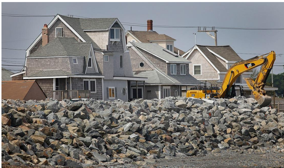
Reconstruction of the Stoney Beach Seawall in Hull, Ma
